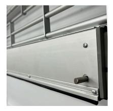
**BOTTOM BAR:** Tubular aluminum extrusion with PVC bulb astragal.
