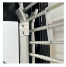
GUIDE ASSEMBLY: Wall angle to be 3/16" minimum thickness structural steel angles. Guides to be extruded aluminum, 3" x 1-1/2" with shoulders for curtain retention fitted with vinyl stripping both sides of curtain with removable headstops.
